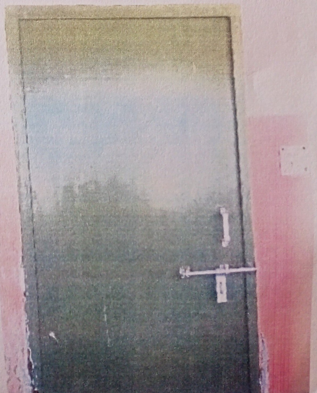
TOILET FOR PERSON WITH DISABILITIES
